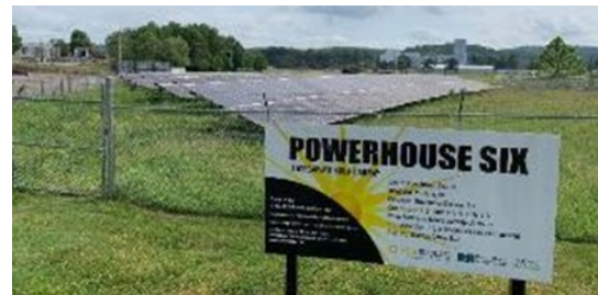
Figure 3.4. Oak Ridge Powerhouse Six Solar Farm
