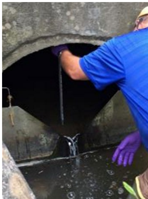
Figure 3.14. Storm water outfall monitoring
