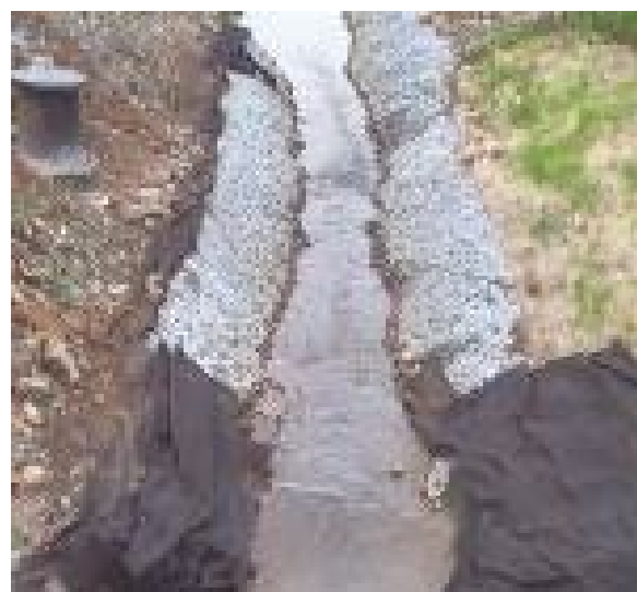
Figure 3.45. Construction of lined section of Mitchell Branch, MIK 0.7, in 1998
